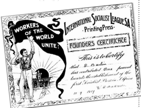
ISL: laying the foundations
